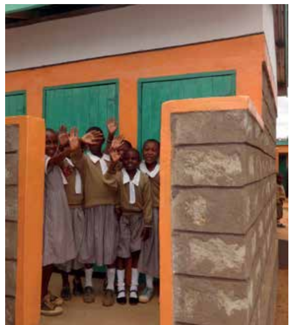
The new latrines at Minyalala Primary School, Machakos
